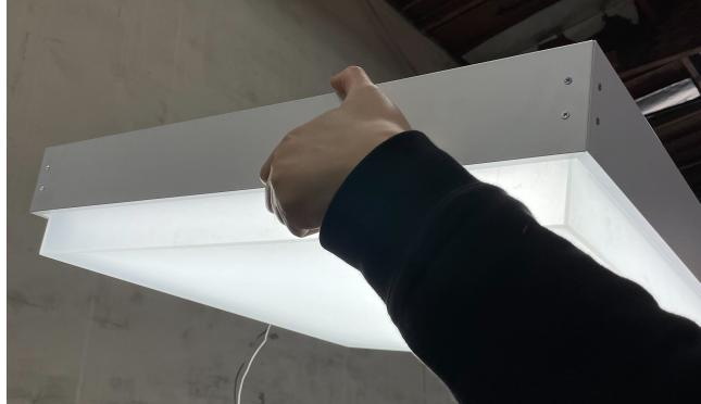
Install the last frame of the SMK to complete the installation.
